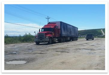
Figure 3: Potholes on highway 510 in Forteau NL, July 2017.
