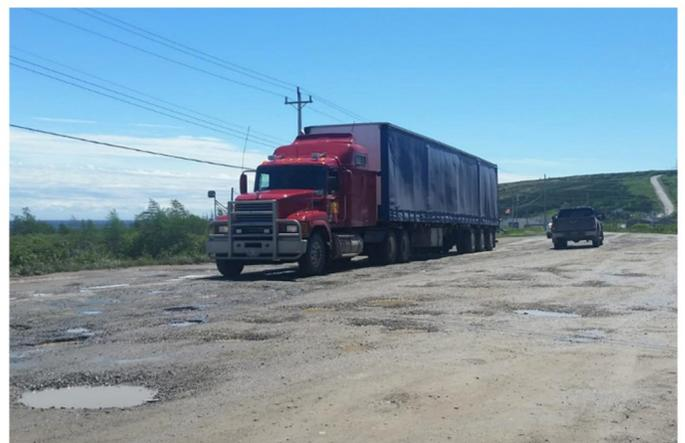
Figure 3: Potholes on highway 510 in Forteau NL, July 2017.
